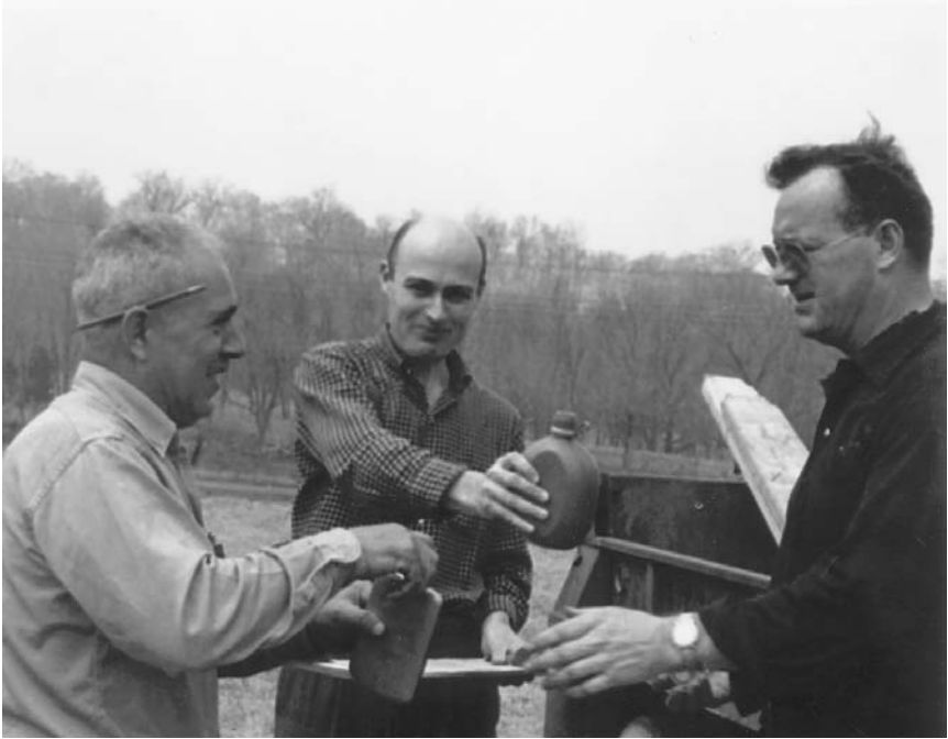
Mills on the construction site of his home in New York, spring 1959. From left to right: Charlie Linguanti, a construction contractor who was Mills's friend and former neighbor, William (Chappy) Diederich, the architect who carried out the Millses' basic design for the house, and Mills. (Photo by Yaroslava Mills.)
